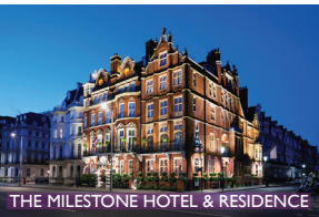
THE MILESTONE HOTEL & RESIDENCE
