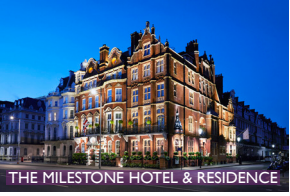
THE MILESTONE HOTEL & RESIDENCE
